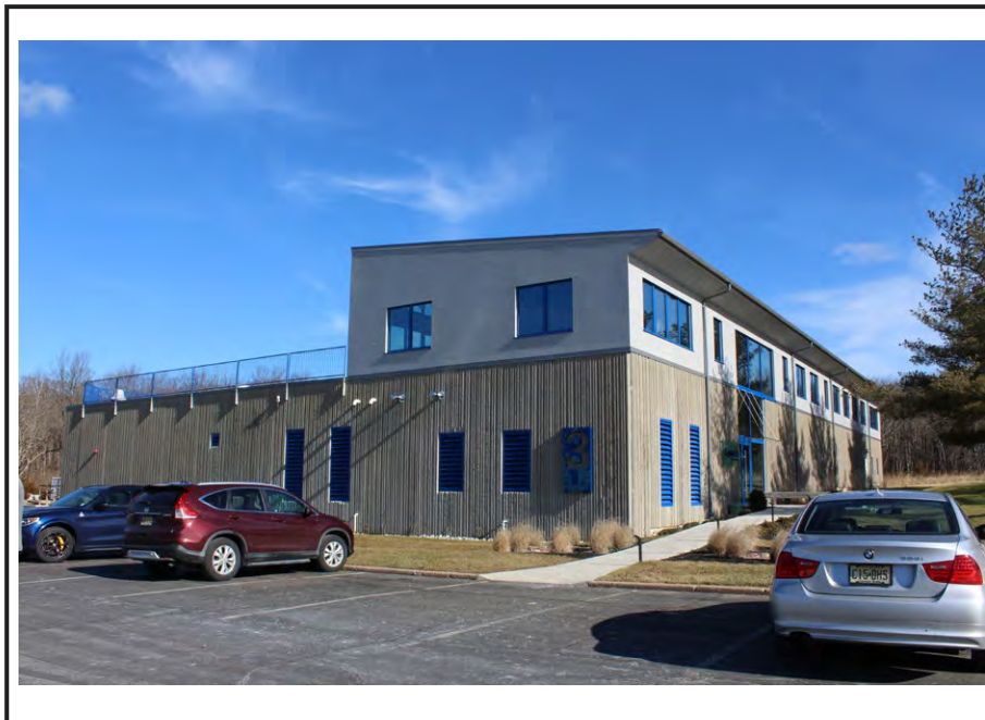
View of the southern corner of the warehouse showing the southeast and southwest elevations. Built south of the substation around 1980, the building consists of a concrete first floor and metal panels on the second floor.
