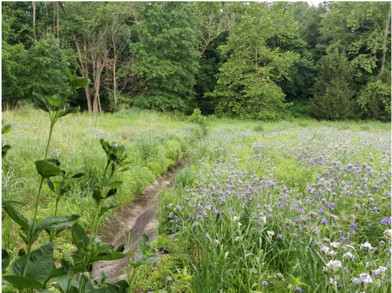
The detention basin low-flow channel stays clear with little maintenance.
