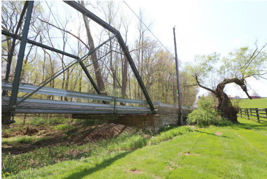
View of the stone abutment and true hanger (tension verticals) located at the northwest end of Bridge 230.3.
