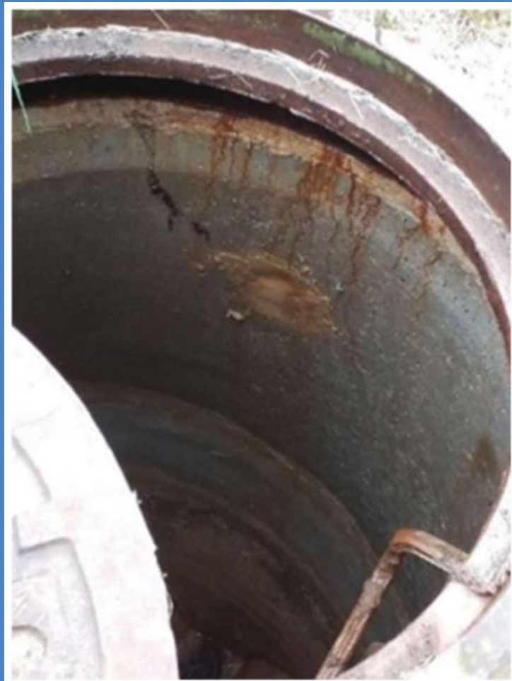
Chimney Infiltration, Staining
