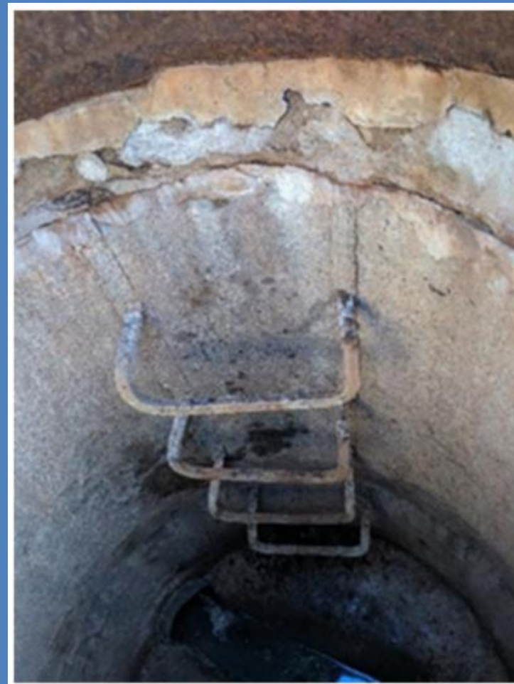
Infiltration, Cracks
