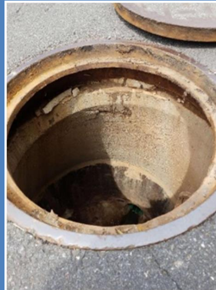
Chimney Loose, Rebar Visible
